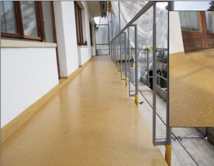
All pictures on this page: terrace/stair/ balcony sealing and coating
