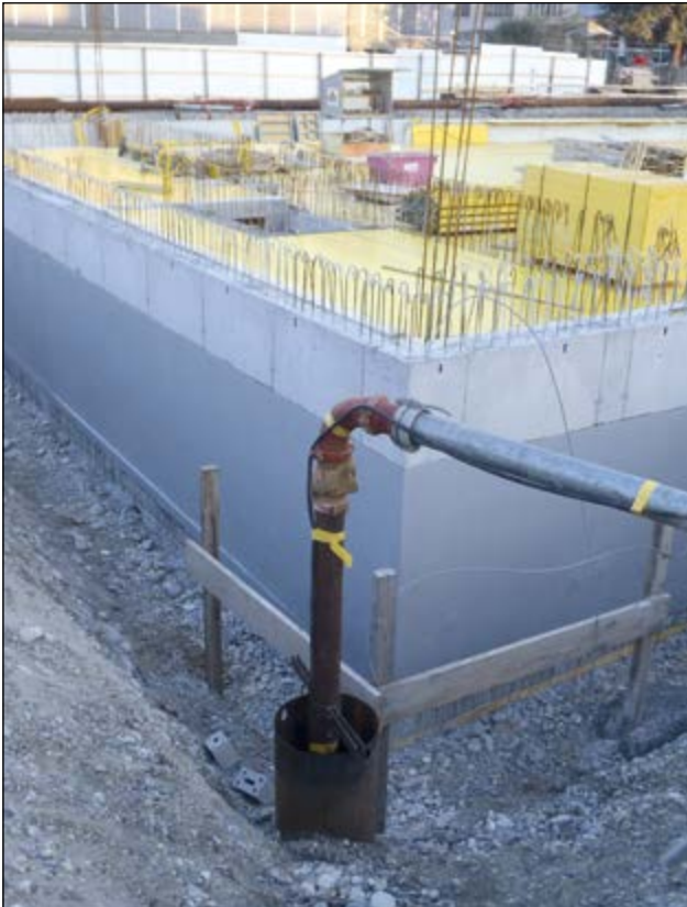
Surface seal in underground area
