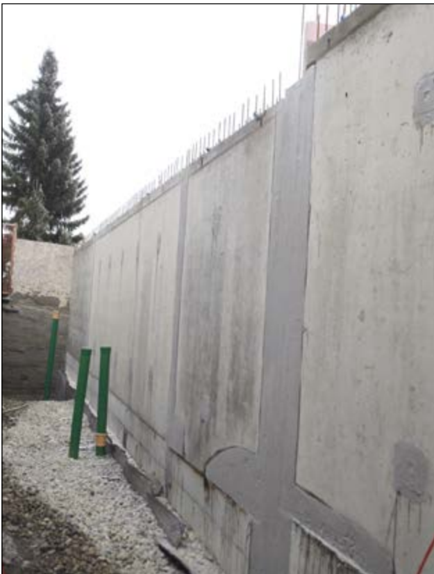
Sealing of construction joints
