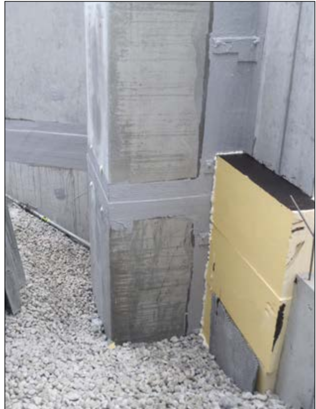
Sealing of concrete construction joints
