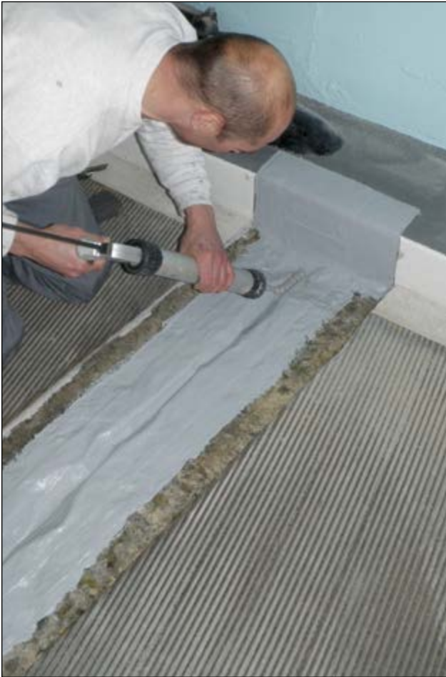
Movement joint/dilatation joint
