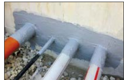
Component connection/surface seal
