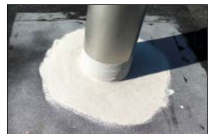
Pipe lead-throughs
