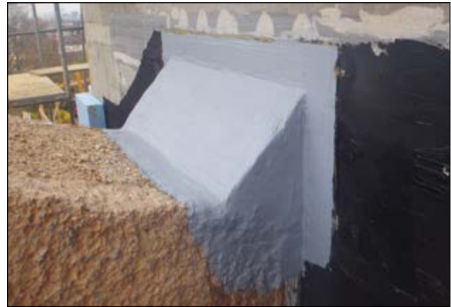
Component connection/surface seal
