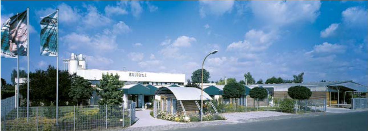
Silikal, production and headquarters in Mainhausen/Frankfurt am Main
