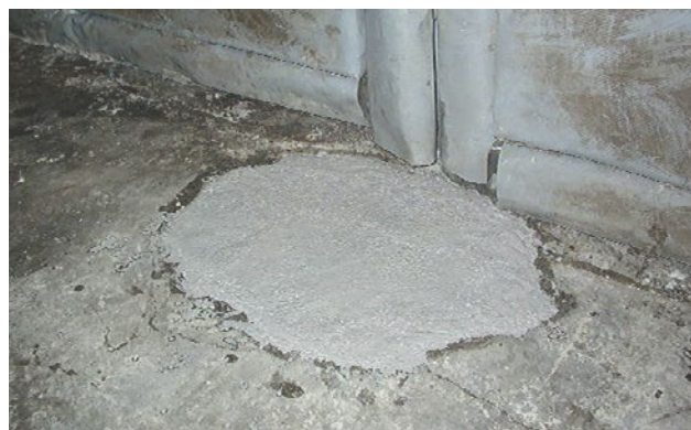
Improvement of the flooring in a cold store in continuous operation with SILIKAL® R 17 (-25 °C) mortar
