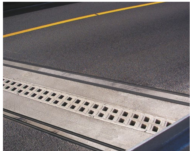
Installation of the lateral drainage channels in a motorway
