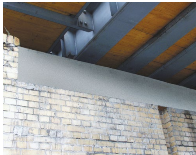
Renovation of the bridge abutment of an urban railway bridge
