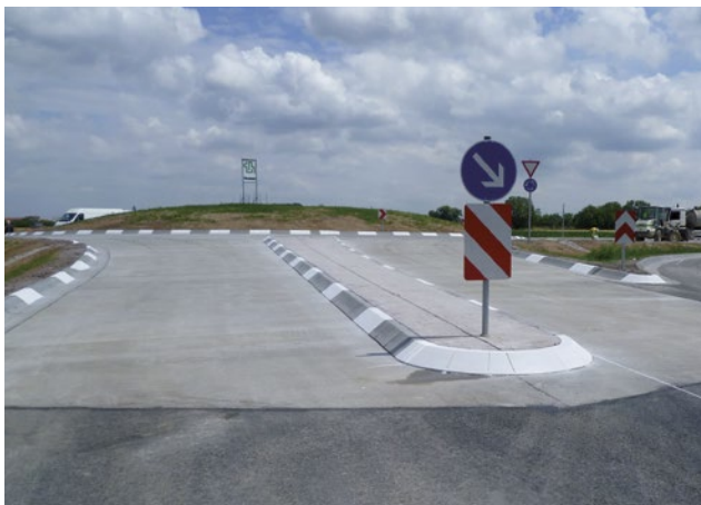
Road renovation of a roundabout with SILIKAL® R 17
