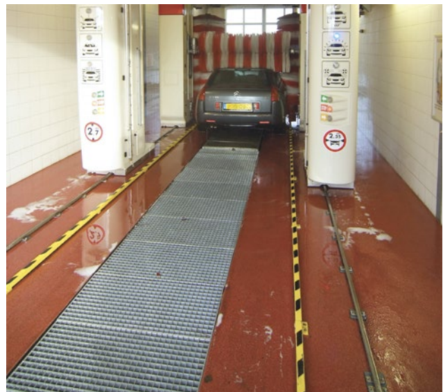
Car wash, Woerden/Netherlands
