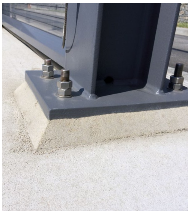
Underlayment of steel construction at an interstate road
