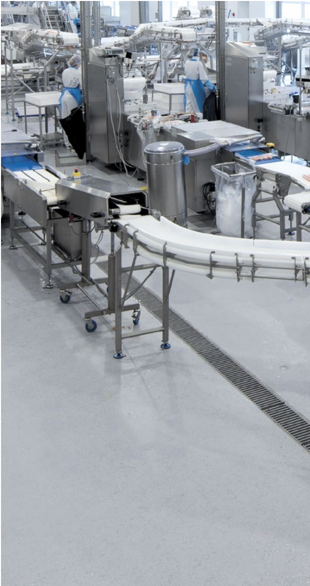
Fish processing facility, Glyvrrar, Faroe Islands
