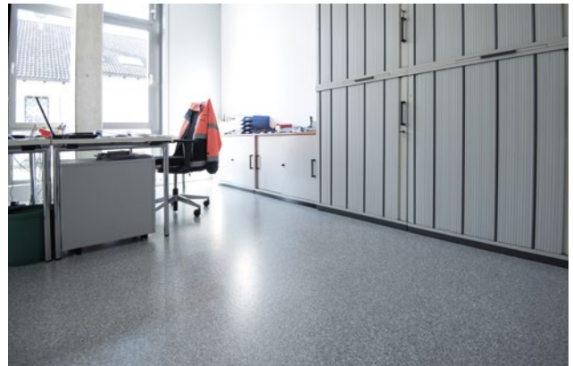
Public utilities, Lohr, Germany
