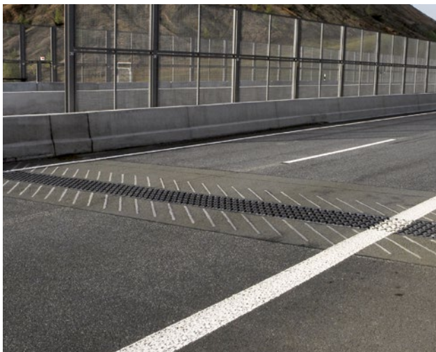
Grouting of supporting ribs in a highway
