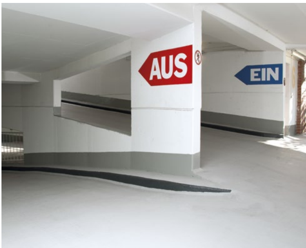
Renovation of ramps in a car park
