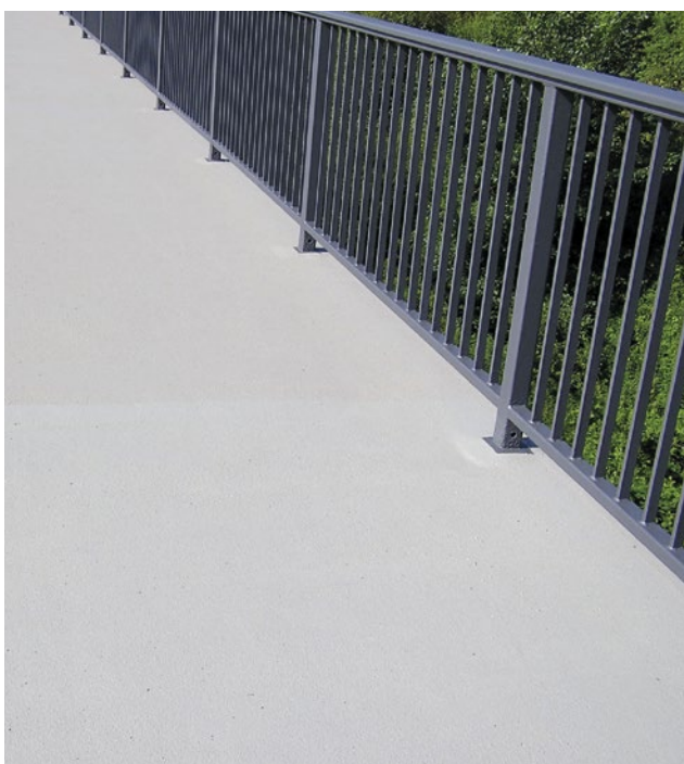
Bridge coating incl. handrail attachment
