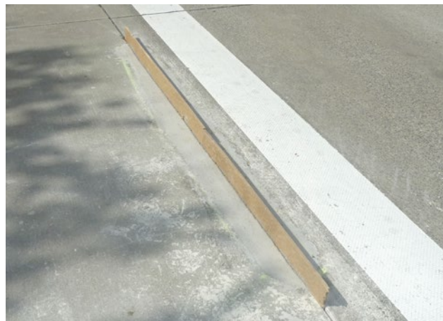
Edge renovation of the concrete roadway of a highway
