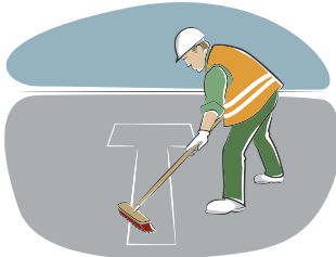
2) Cleaning of the surface
