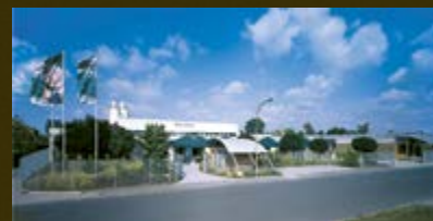
Silikal production and administration in Mainhausen, near Frankfurt/Main, Germany.
