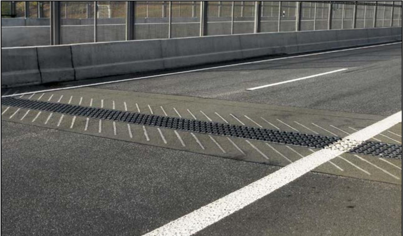
A38 Motorway near Breitenworbis/Germany: Joint rip profile installation
