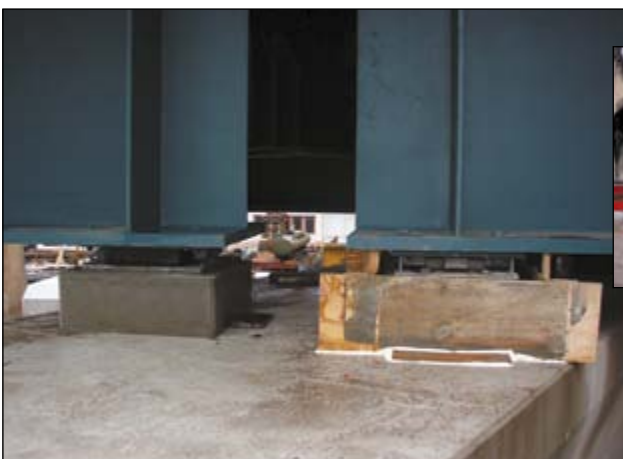
Chemnitz-Einsiedel viaduct, Blankenauer street: repairing bridge bearings
