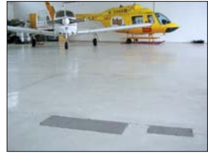
Mannheim Airport Repairing hangar floors
