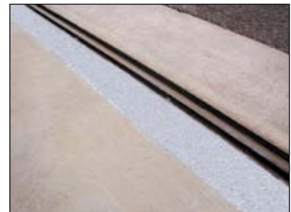
Mannheim Airport: Laying foundations of sliding door rails
