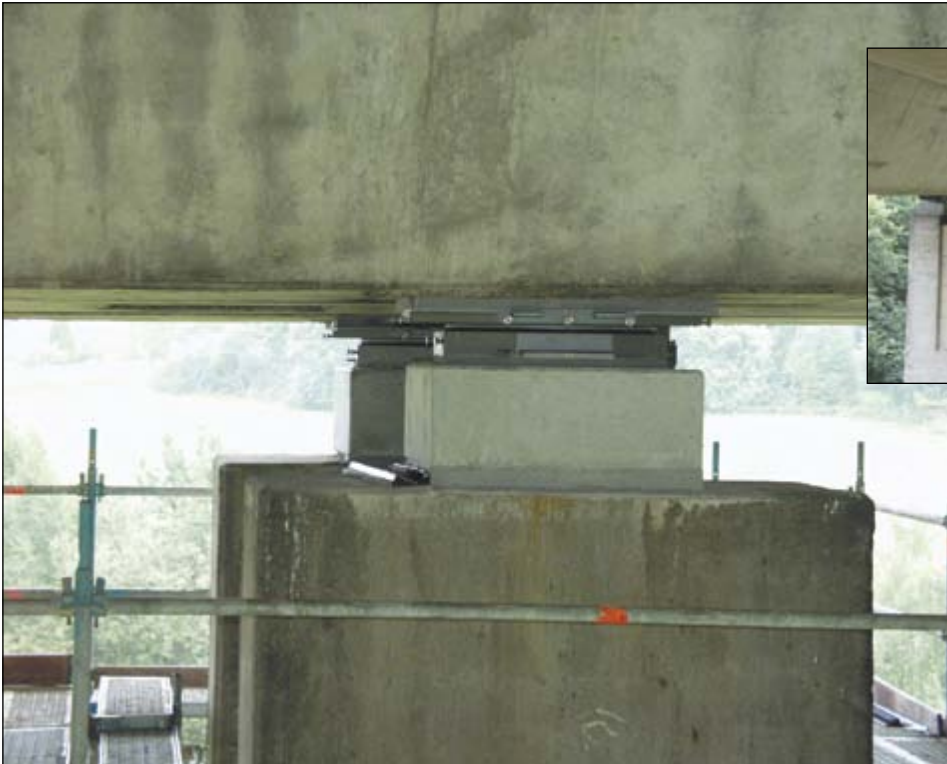
A7 motorway bridge, Uttrichshausen: Repairing bridge bearings
