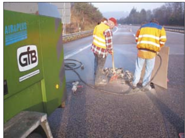
A3 Motorway, Neustadt/Wied: Improving the road surface
