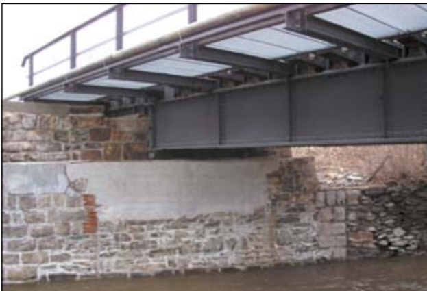
Chemnitz-Einsiedel viaduct, Blankenauer street: repairing bridge bearings
