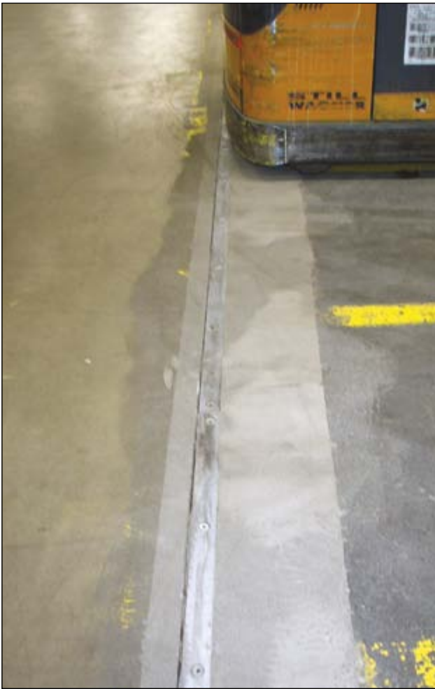
Metro AG, Essen: Renovation of expansion joints in a warehouse
