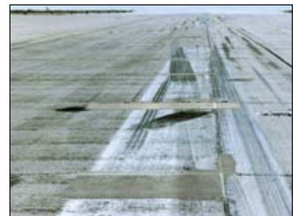
Leipzig/Halle Airport: Repairing concrete, runways and taxiways
