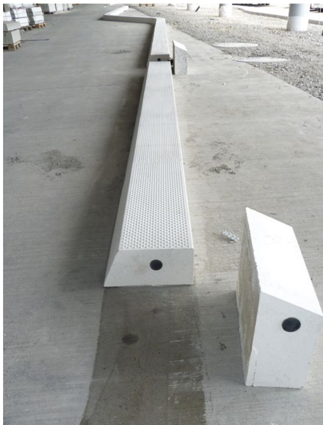
Car park airport, Stuttgart/Germany: Kerb stone stuck to concrete with SILIKAL® R 17-thix
