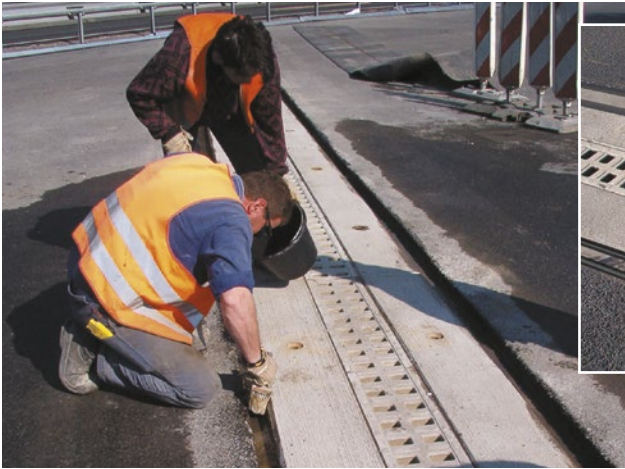
A2 Motorway, Hamm-Uentrop/Germany: Construction of transverse drainage channels
