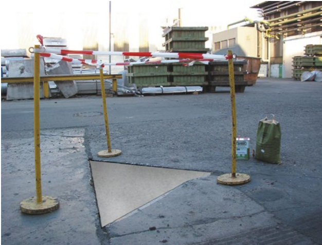
CORUS aluminium rolling mill, Koblenz/Germany: Repairing traffic areas
