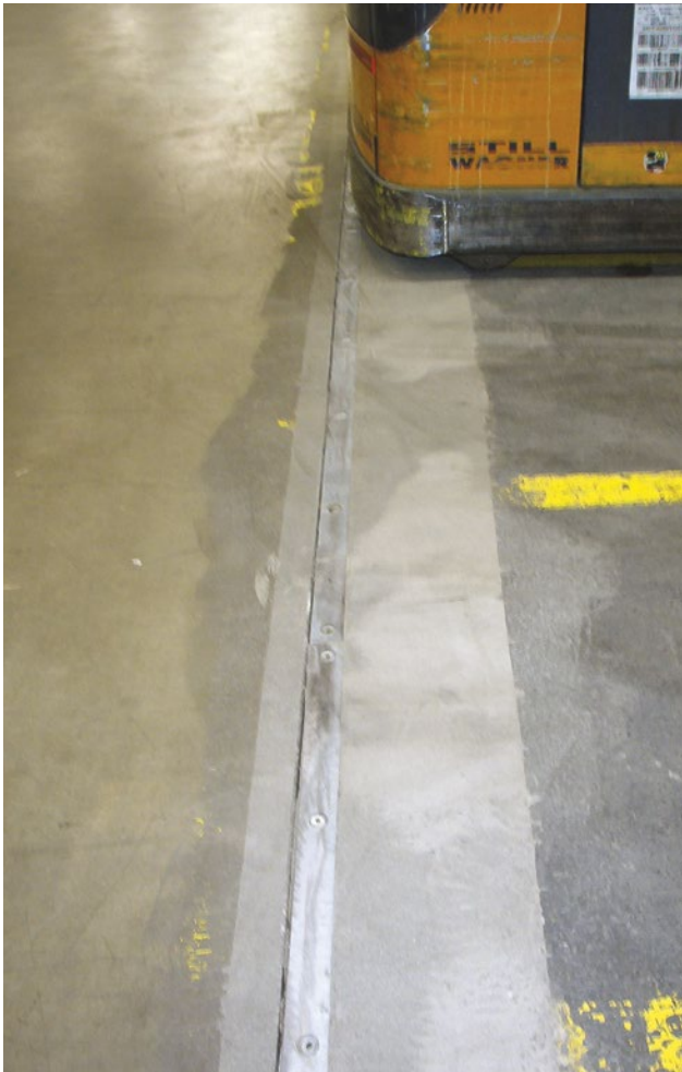
Metro AG, Essen/Germany: Renovation of expansion joints in a warehouse
