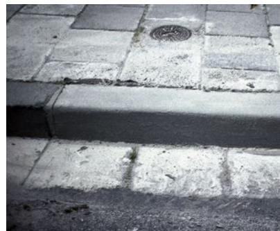
Repairing the kerbs with SILIKAL® R 17
