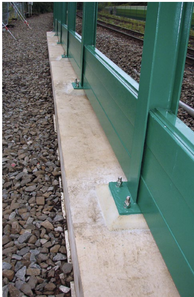
Railway track Koblenz-Bonn/Germany: Underlayment of steel columns for noise protection
