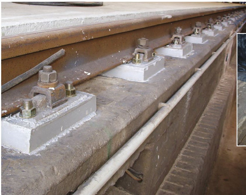
Deutsche Bahn AG, Braunschweig railyard/Germany: Renovation of track storage
