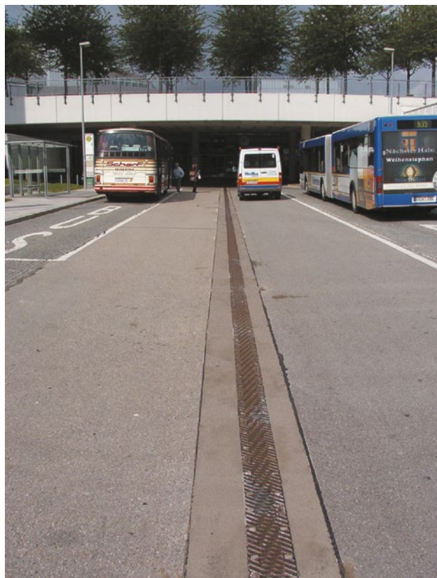
South bus station of the "Franz-Josef Strauss" airport, Munich/Germany: Repairing drainage channels
