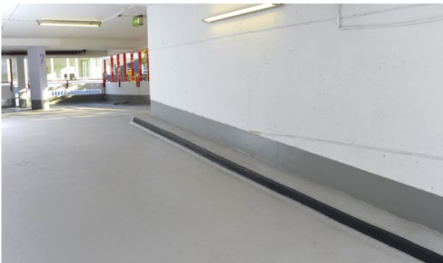
Car park "Altlohrtor", Koblenz/Germany: Renovation of ramps
