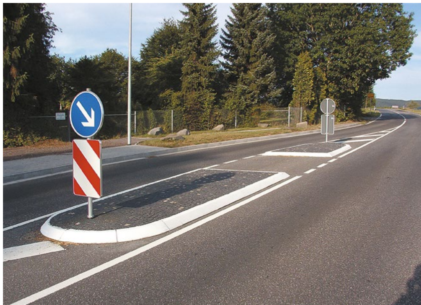
K 106 by-road, Neuwied-Niederbieber/Germany: Kerb of a traffic island stuck to the asphalt with SILIKAL® R 17
