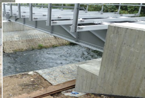
New railway bridge construction in Grafenwöhr/Germany: Bridge bearings
