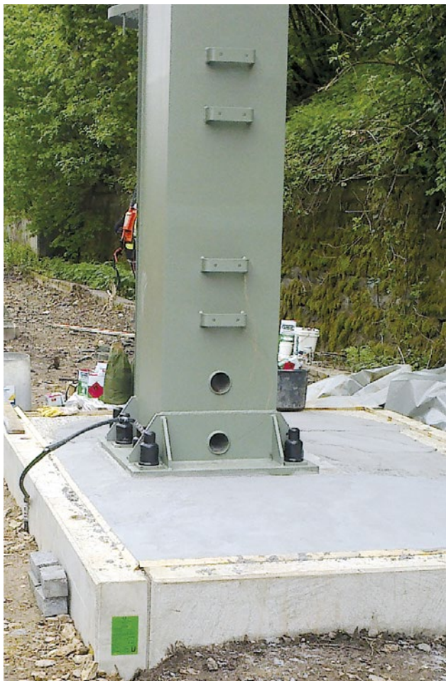
Railway track Düsseldorf-Wuppertal/Germany: Installation of steel columns
