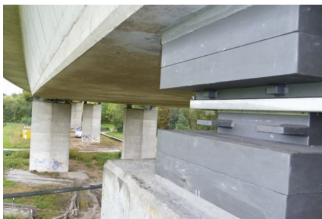
A6 Motorway Bridge, Massholdertal/Germany: New bridge bearings
