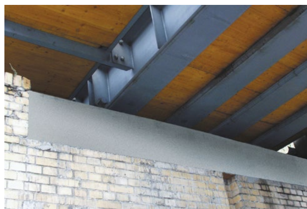
Metropolitan viaduct, Berlin/Germany, Sterndamm: repairing bridge bearings
