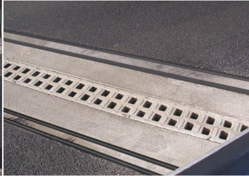
A2 Motorway, Hamm-Uentrop/Germany: Construction of transverse drainage channels
