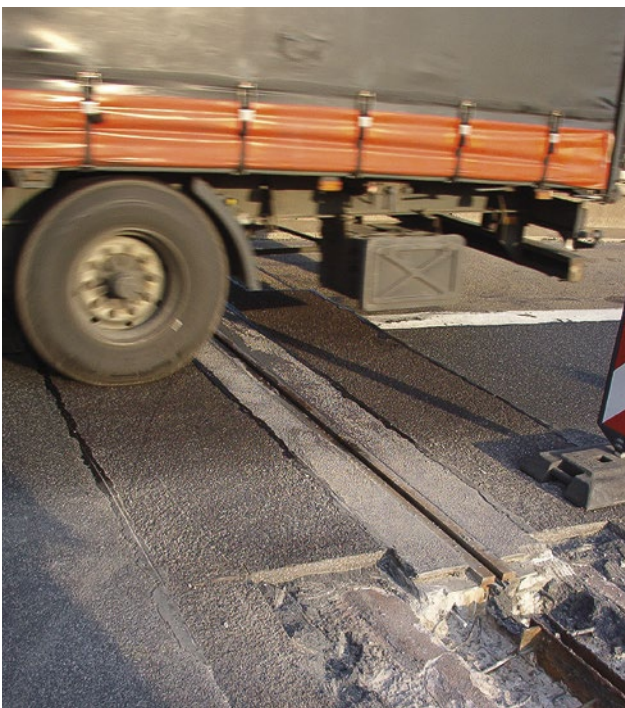
A45 Motorway near Solms/Germany: Repair and implantation of joint profiles
