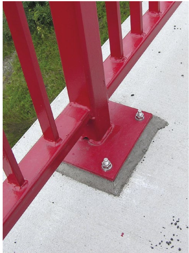
River Rhine Bridge near Wesel/Germany: Underlayment of hand rail columns
