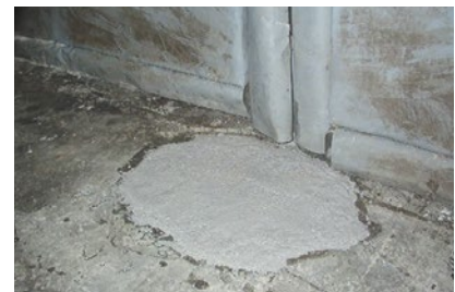
Figure on top: Deutsche See GmbH & Co. KG, Bremerhaven/Germany: Repair of floor areas in cold store house with SILIKAL® R 17 with no disruption to operation (-25 °C)
