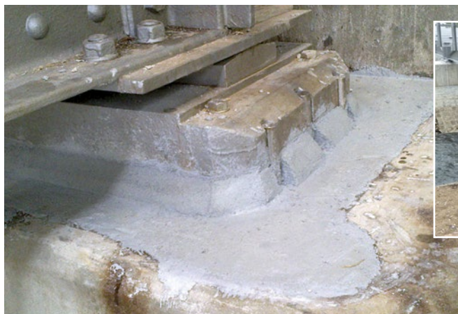
A6 Motorway Bridge, Massholdertal/Germany: New bridge bearings
