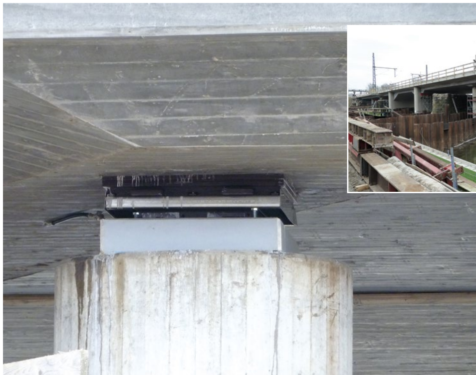
New railway bridge construction in Hannover-Ohedamm/Germany: Bridge bearings
