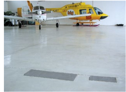
Mannheim Airport/Germany: Repairing hangar floors
