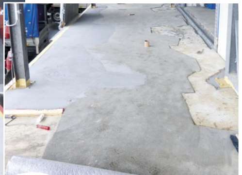
Forwarder warehouse, Kassel/ Germany: Renovation of a loading ramp
