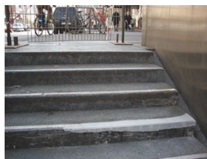
Metro station stairs in Venloer street, Cologne/Germany: Repairing the steps
