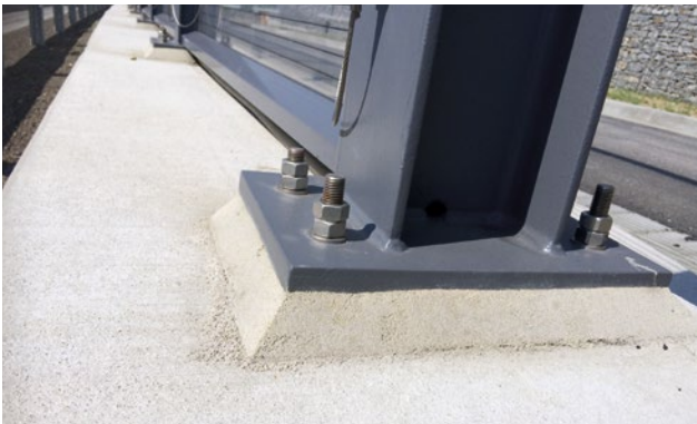
B42 Interstate Road/Germany: Underlayment of steel construction
