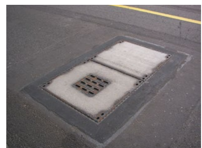
Nordrhein-Westfalen Airport/Germany: Sealing cable ducts with asphalt- coloured SILIKAL® R 17
